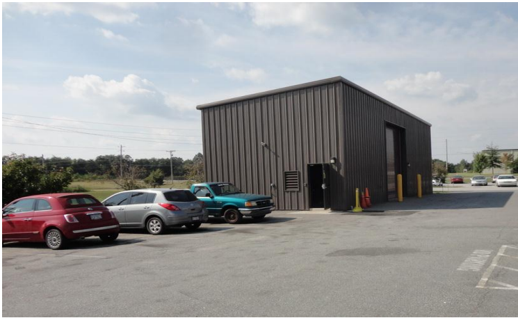
View of Waste Water Treatment Building (2007)
