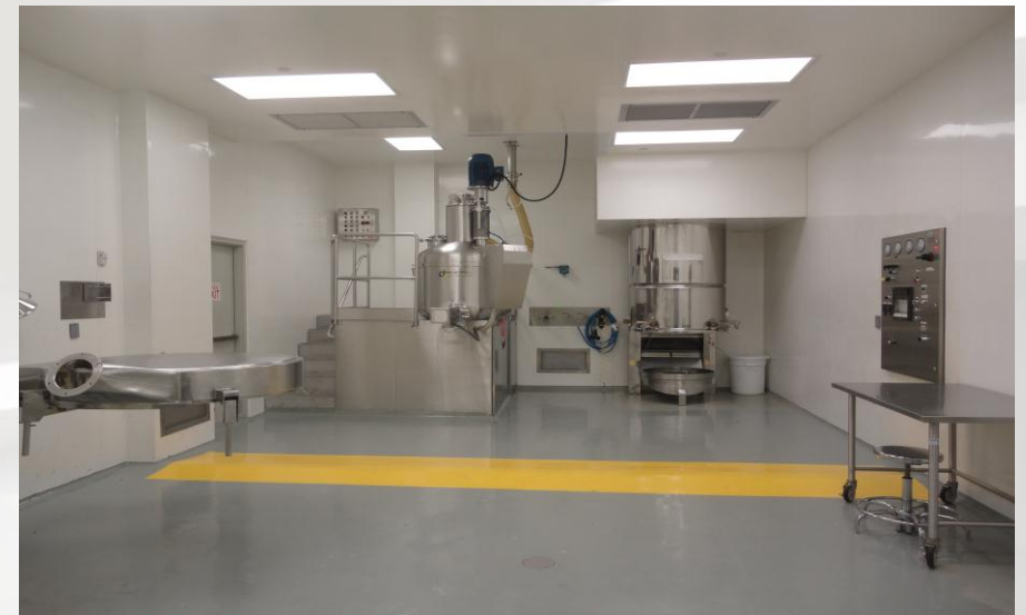
View of Production Suite with Zanchetta 400 liters High Shear Granulator with Aeromatic Fluid Bed Dryer
